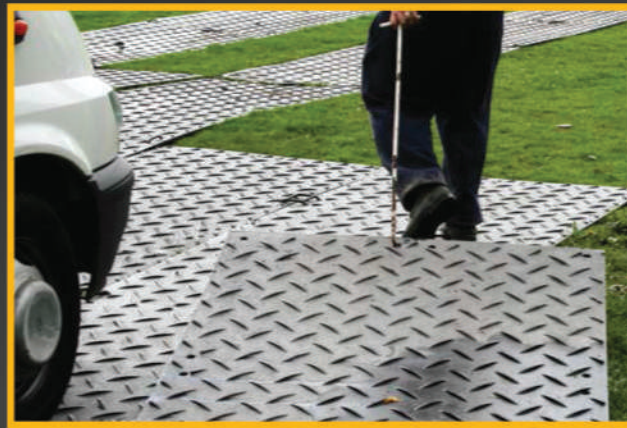
The Handi Hook enables easy moving of mats on site
